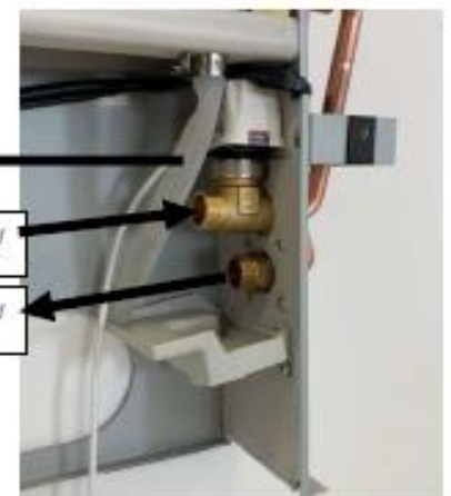
PUT INSULATION IN ALL THE EXTERNAL PIPE
