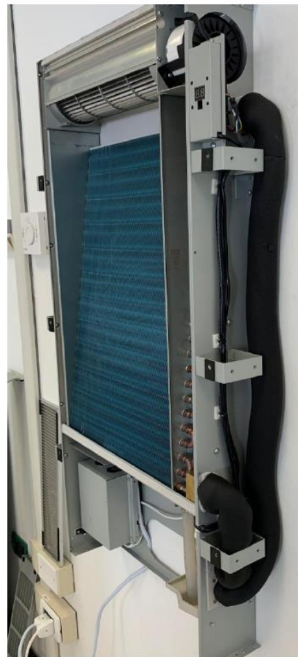
PUT INSULATION IN ALL THE EXTERNAL PIPE
