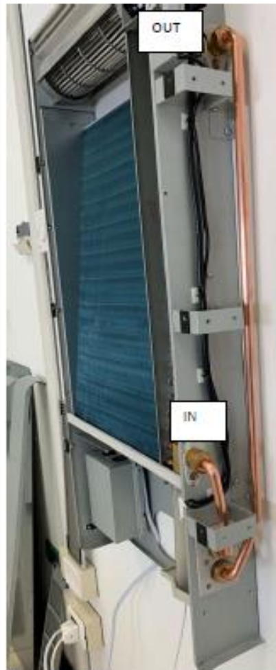
PIPE CONNECTION WITHOUT INSULATION
