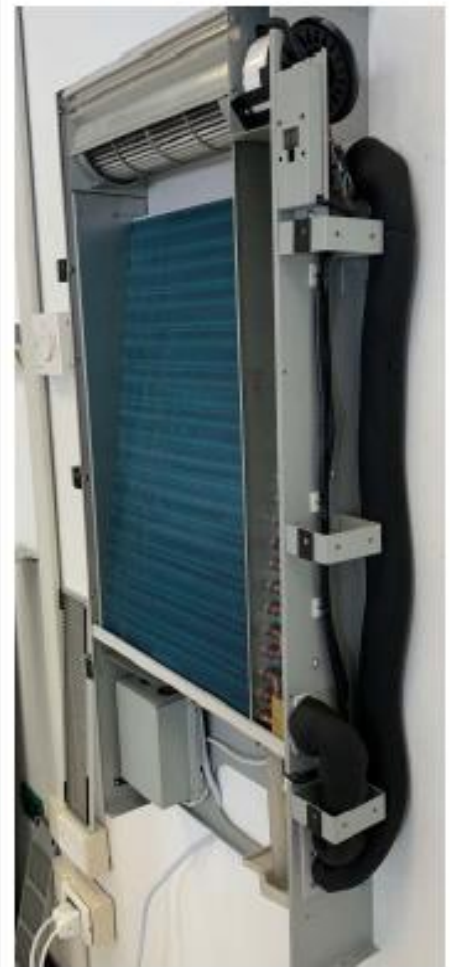
PUT INSULATION IN ALL THE EXTERNAL PIPE
