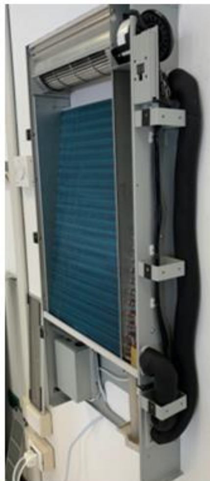
PUT INSULATION IN ALL THE EXTERNAL PIPE
