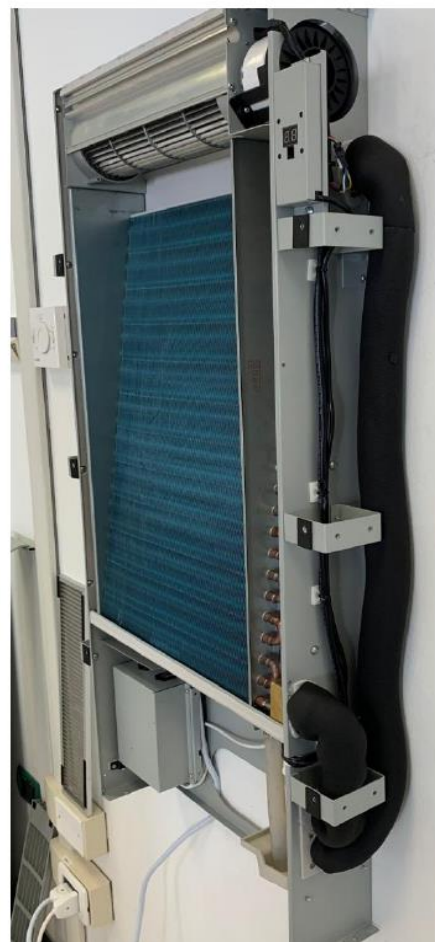
PUT INSULATION IN ALL THE EXTERNAL PIPE
